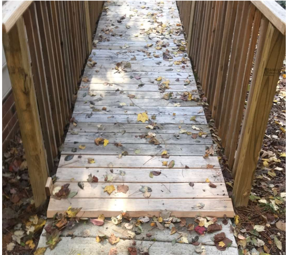
Back of the House Ramp Entrance (Ramp 2)
