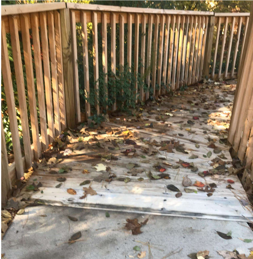
Back of the House Ramp Exit (Ramp 2)
