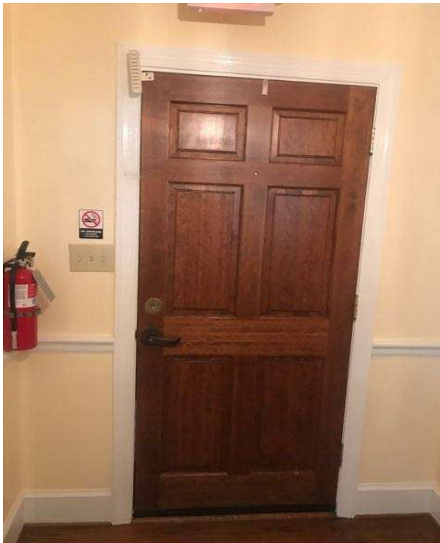
Front Door Entrance view from Front Entrance Hallway
