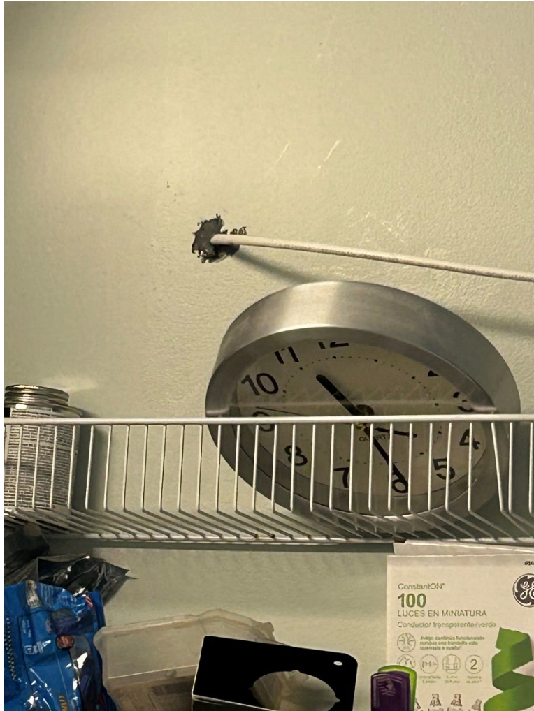
Fireproof caulk sealing cable hole in room 13
