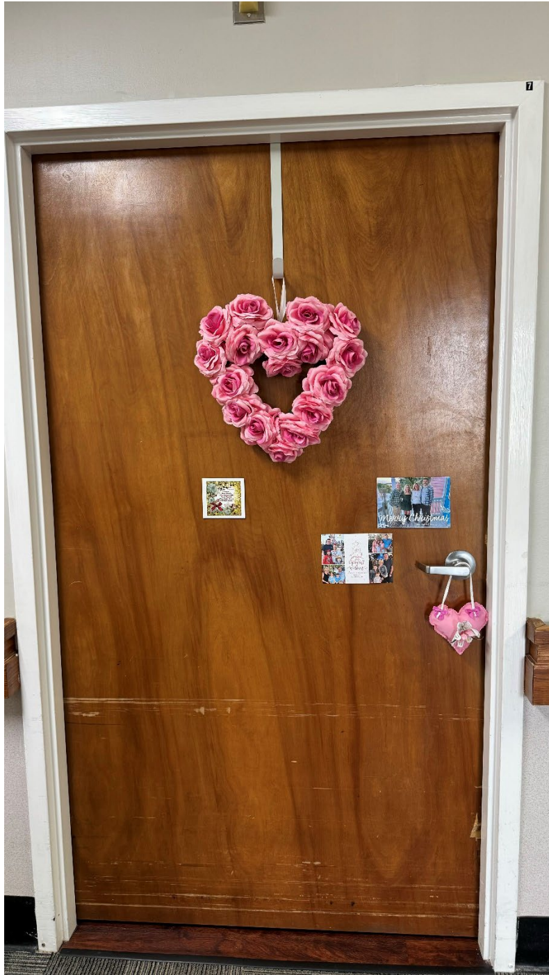
Room 7 has been repaired and now latches when the door is closed.
