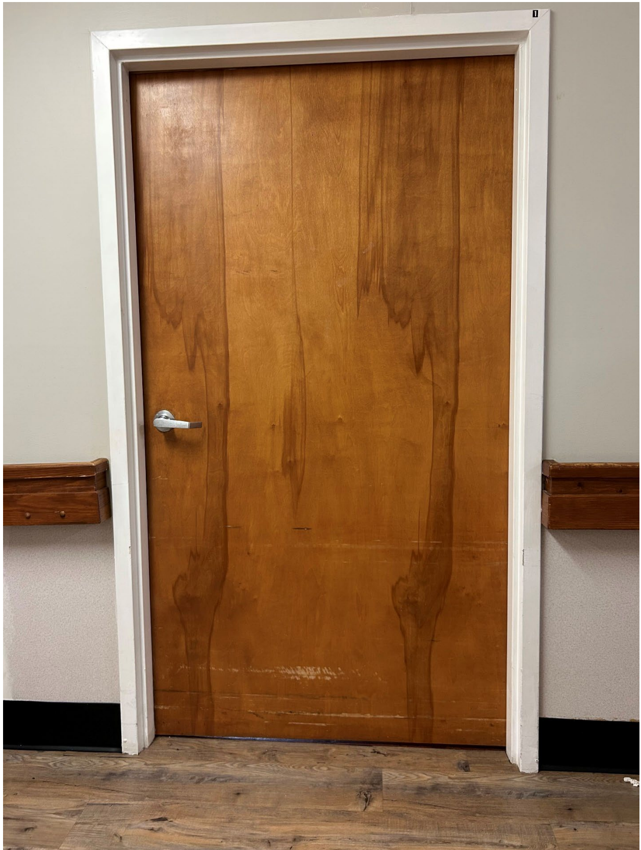
Room 1 repaired to remove 1/2" gap at the top left of the door between the door and the door frame.
