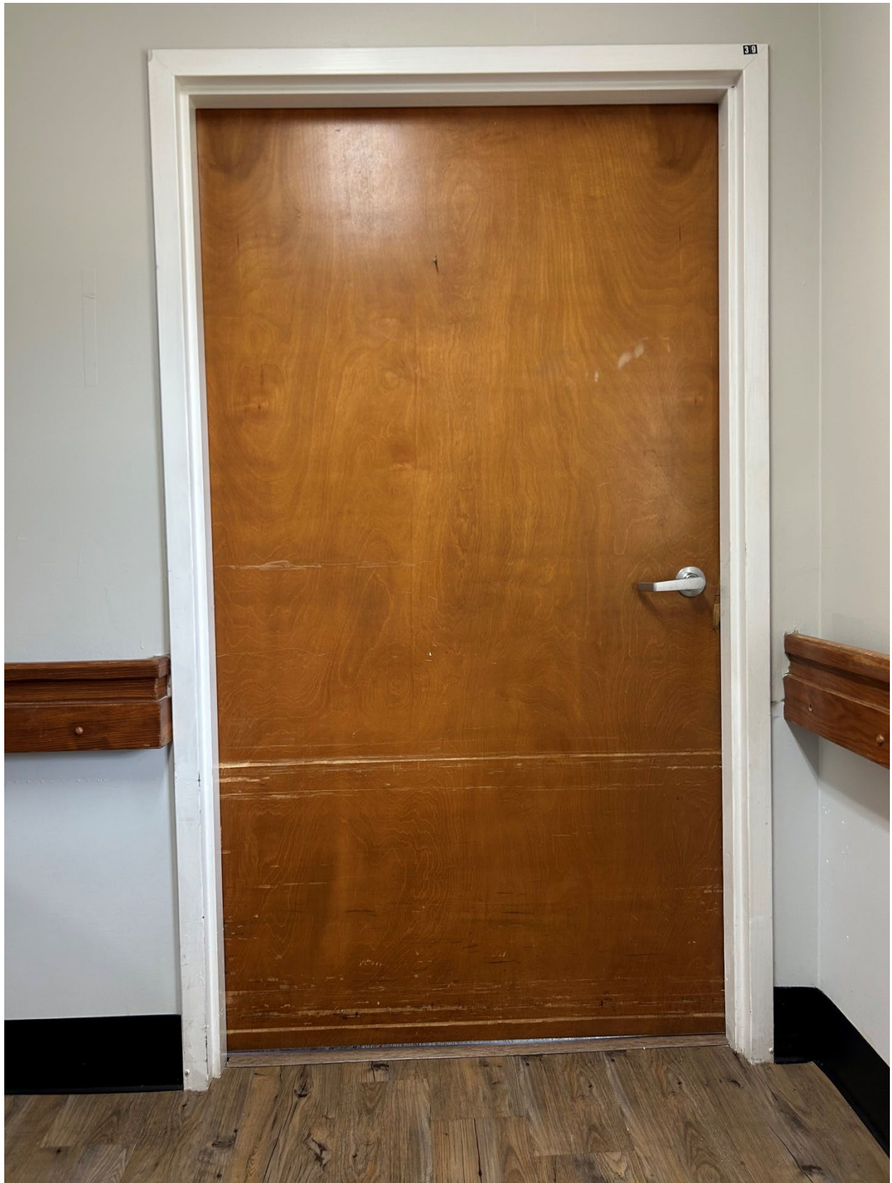
Room 39 repaired so that the door is no longer hitting the threshold, closes and latches.
