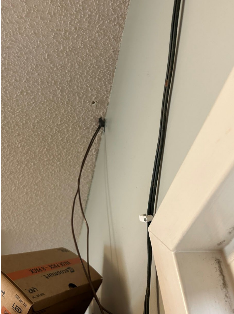
Fireproof caulk sealing cable hole in room 13
