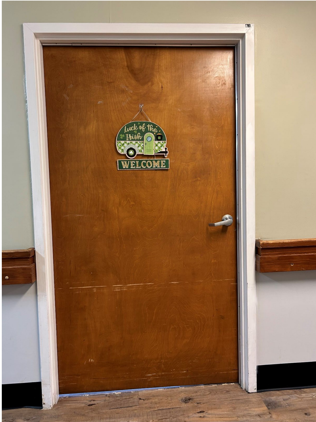
Room 41 repaired so that the door is no longer hitting the threshold, closes and latches.
