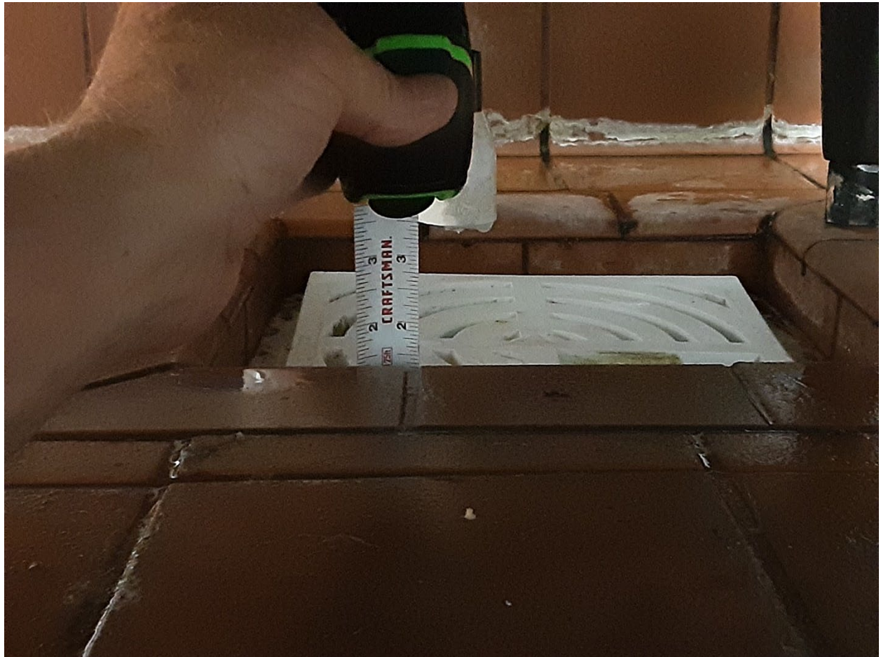
Kitchen drain space
